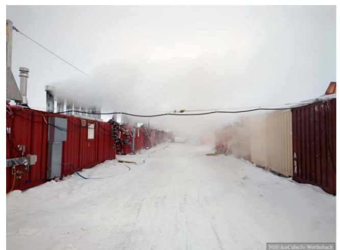
View to the drill cap with the heaters working to warm up the water for the drill.
