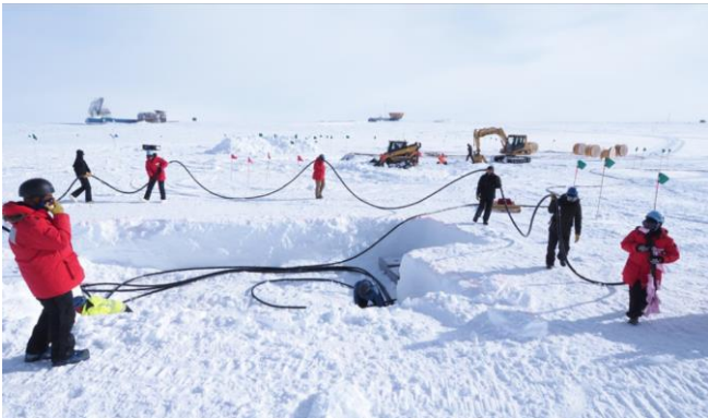
Coiling the surface cable slack into the pit required all hands on deck. A string anchor is being installed in the background (Photo. C. Hill)
