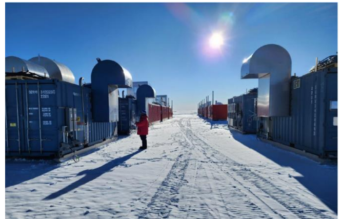
Top: View of "Seasonal Equipment Site" (SES) with the IceCube Laboratory in the background. In the foreground are the main heating plants. Bottom: view down the aisle of the SES showing the generators in the foreground, water tanks and main heating plants in the distance. (Photo: K. Studt, IceCube/NSF)
